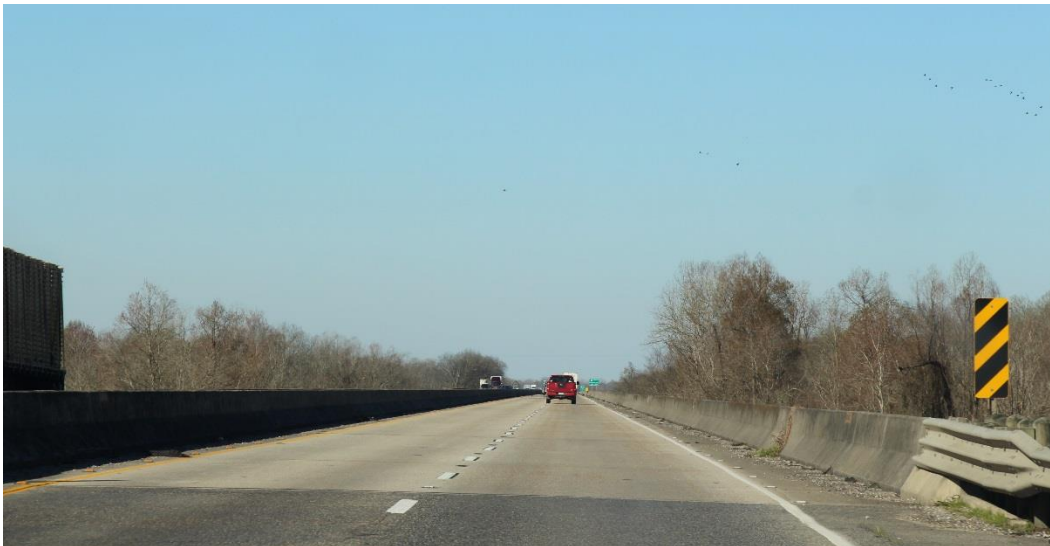
Condition Photo 17: East roadway approach looking west.
