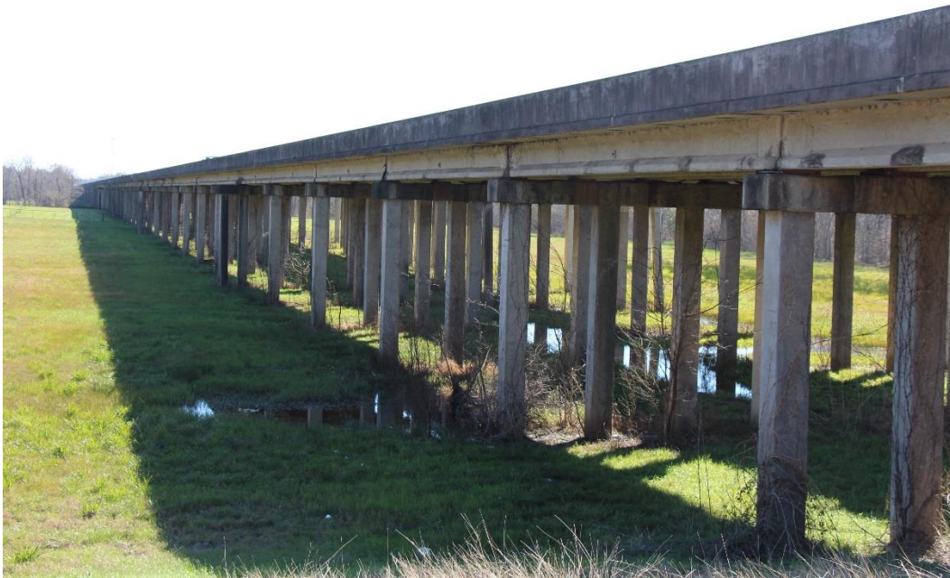
Condition Photo 18: Elevation view looking east.
