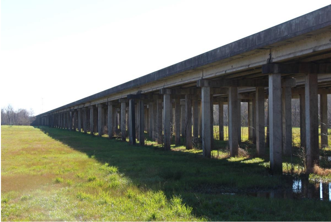
Character-defining Feature Photo 1: Prestressed concrete girder superstructure (Recall No. 007300).
