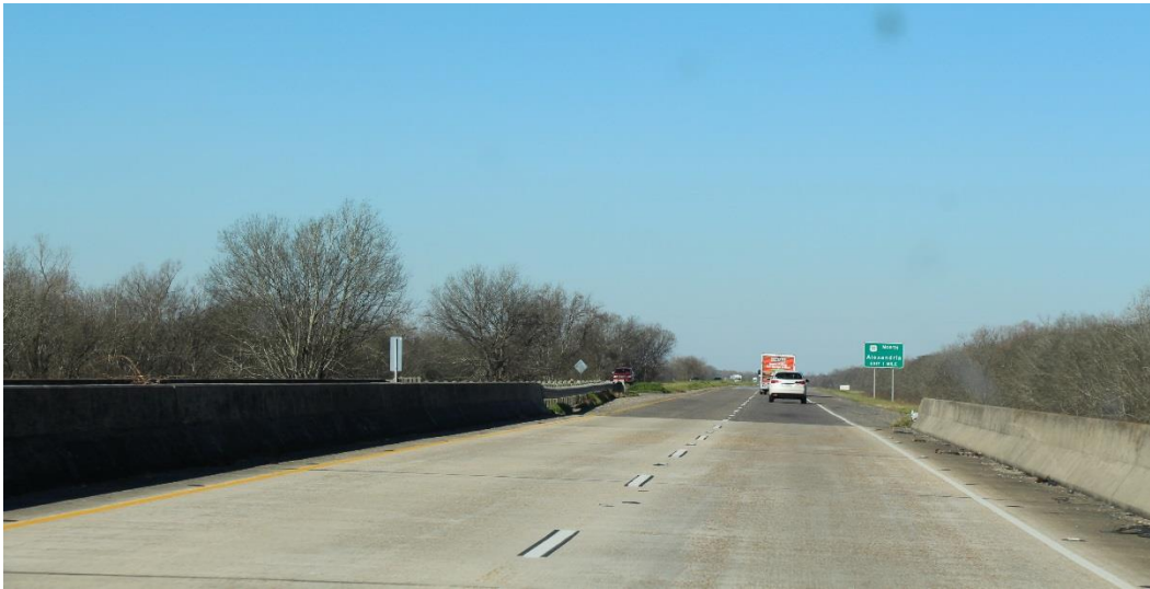
Condition Photo 16: West roadway approach looking west.
