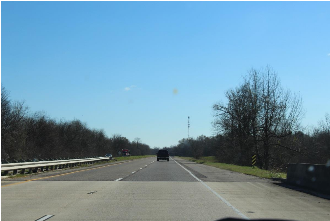
Condition Photo 1: West roadway approach looking east.
