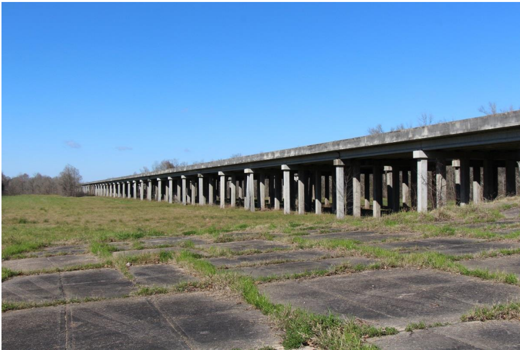
Condition Photo 3: Elevation view looking west.
