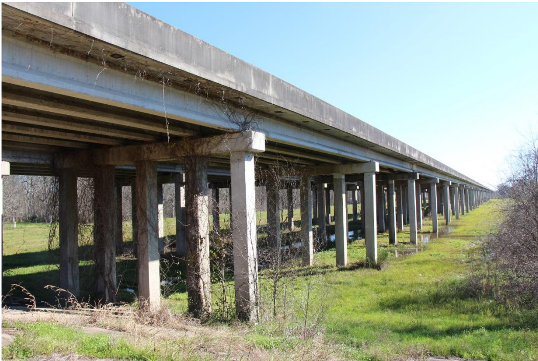
Character-defining Feature Photo 2: Prestressed concrete girder superstructure (Recall No. 007310).
