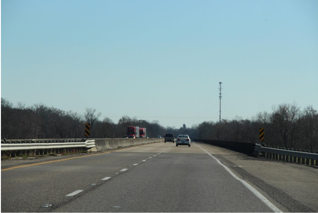
Condition Photo 2: East roadway approach looking east.
