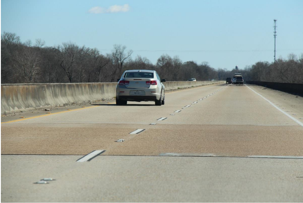
Condition Photo 4: Typical top of deck roadway surface looking east.
